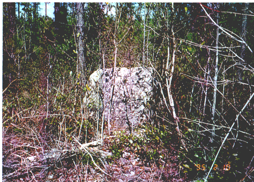
J-18 Area E: Range XX; foundation for observation tower that was removed from road; see plate 8.
